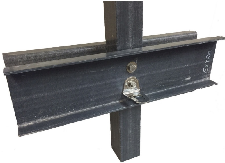
3107-1 Anchorage Connector Installed to Fiberglass Cooling Tower Structure
